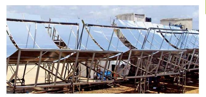
The SharperSun Space Frame was specially designed to reduce the assembly time on the ground and reduces auxiliary power consumption, besides being durable and corrosion-resistant. The SharperSun team is now working on an innovative single-axis tracking system that significantly reduces auxiliary power consumption required for tracking.
